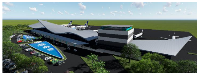
Figure 11. Application of metal sheet roof material
