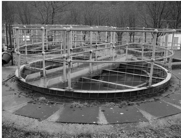
Fig no.4.1 Primary Sedimentation Tank
