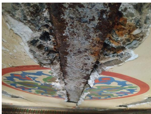
Image (5) shows The spread of rust in iron beams and roof concrete
