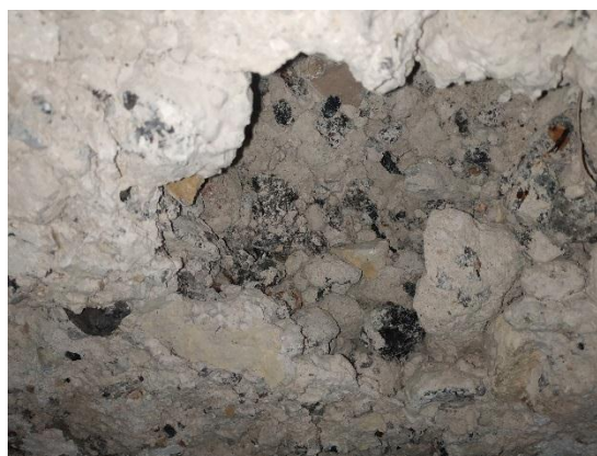
Image (9) shows Details of the location of the loss of concrete (the concrete sample that was studied)
