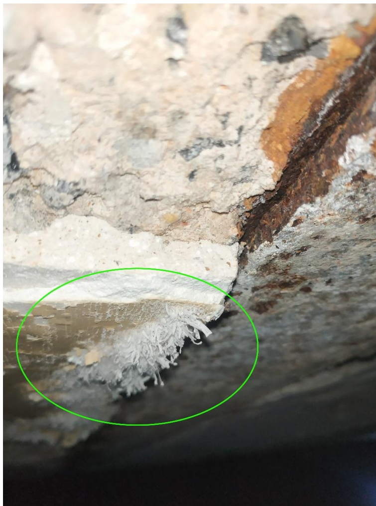
Image (7) shows render layers damage and the salts efflorescence on the color layer Surrounded by the green circle, the salt sample was taken from these salts efflorescence
