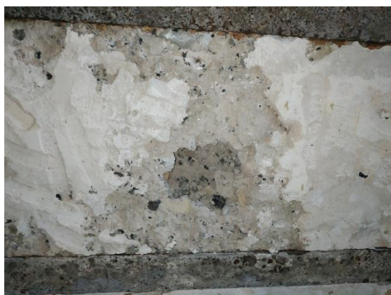
Image (8) shows Parts of concrete falling
