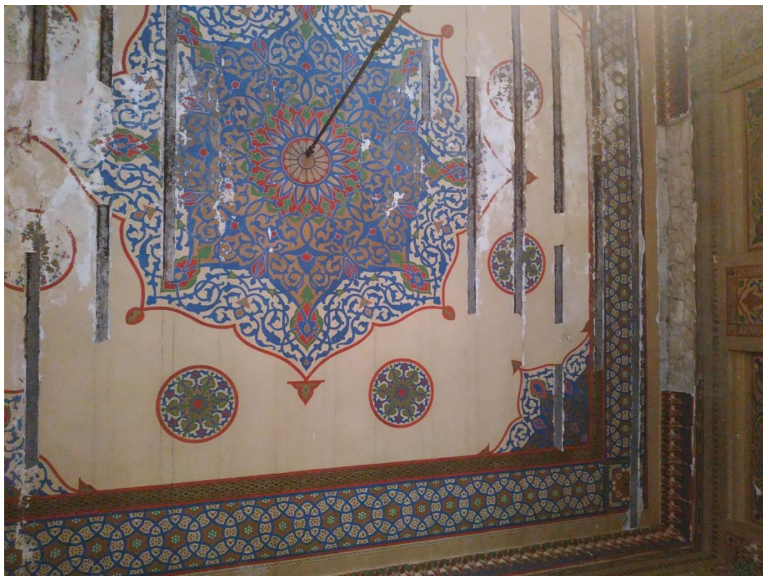
Image (4) shows the ceiling slab damages in the decoration area
