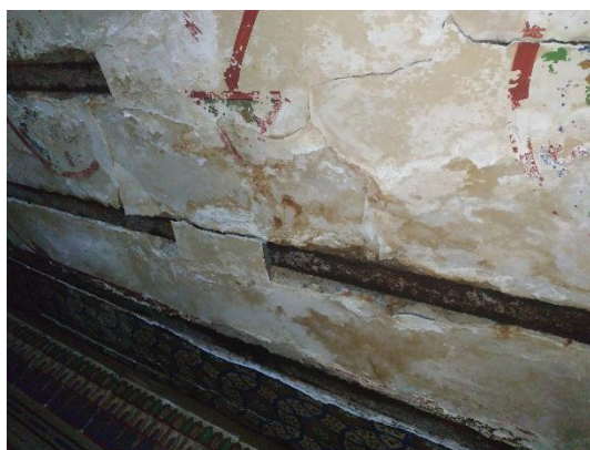
Image (6) shows peeling of colors, separation of render layers, and the spread of cracks
