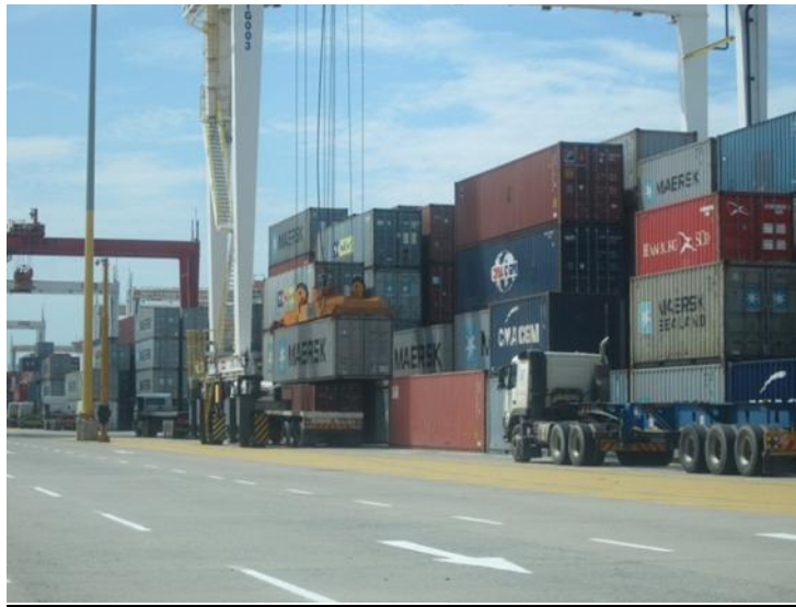
Figure 2: RTG operation- DCT Pier 1
