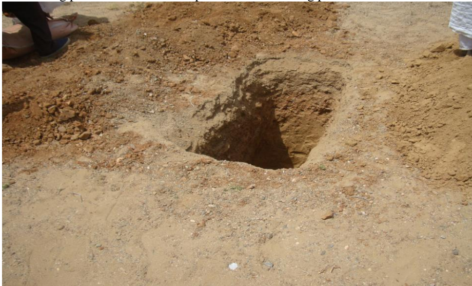
Figure (1): soil Testing Pit
