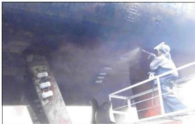
Figure 8 – Blasting with pressurised water and installation of zinc anodes
