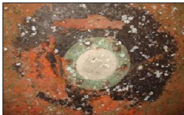
Figure 6 – Insulated support of inert anodes
