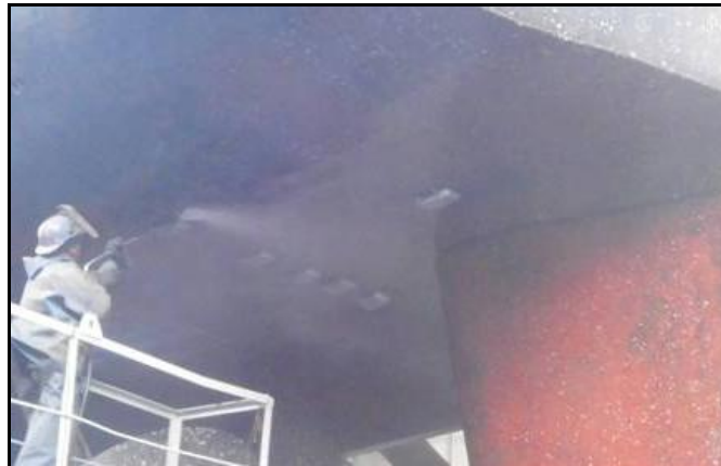
Figure 7 – Blasting with pressurised water and installation of zinc anodes
