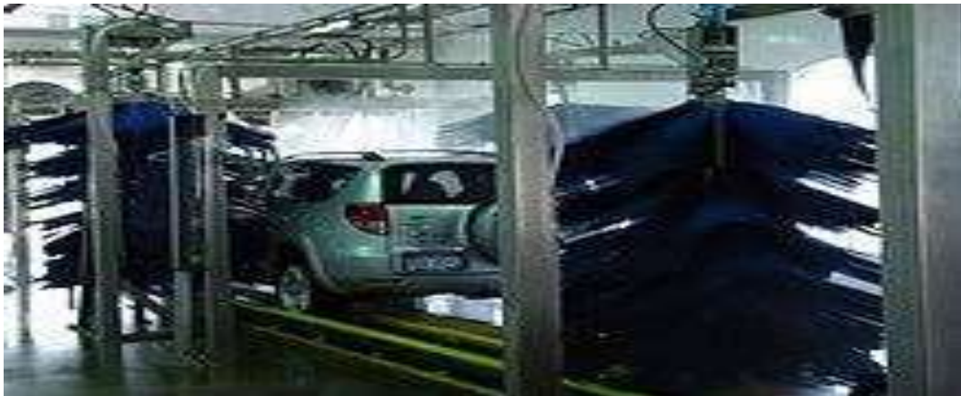
Fig. A vehicle in the high pressure rinse stage of the wash.
